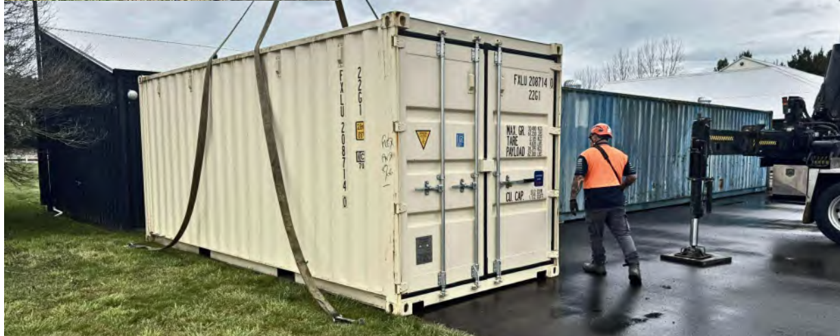
New Emergency Container installation at marae
